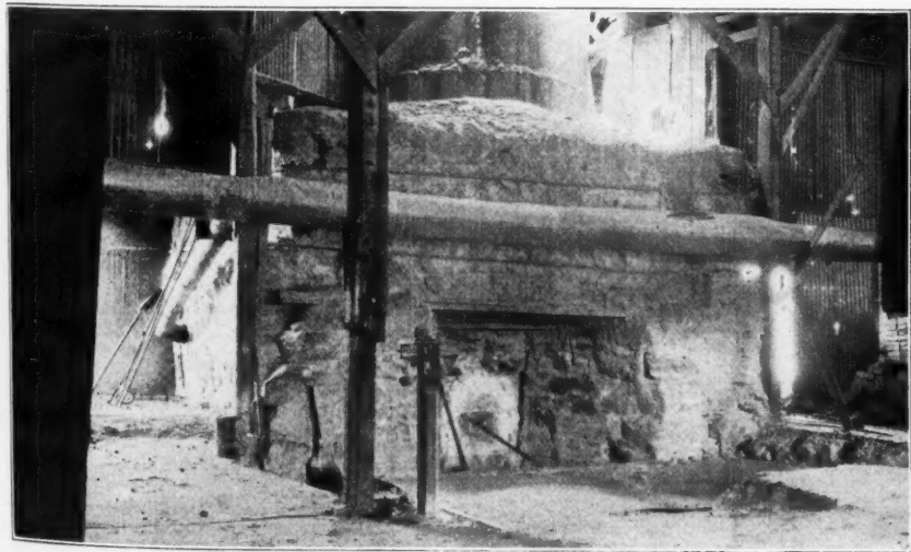
Interior Showing Base of Kilns and Flues for Forced Draft.
